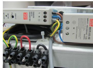
Figure 4: 48 VDC Power Supply
